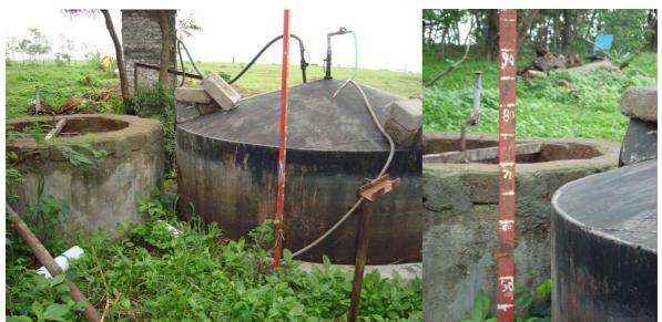
Using the measuring stick next to the gas holder note down the reading before and after every feeding, and enter these numbers into columns 4 and 5.
