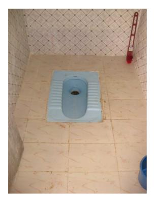
If the W.C doesn't have a flush mechanism it is important that we remember to install a tap so that the user can manually flush the W.C.
